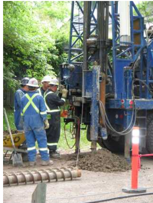
Monitoring well abandonment 2008.
