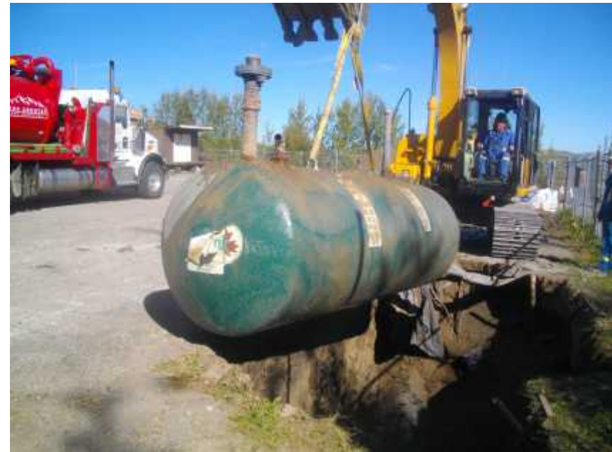
Example of an Underground Storage Tank Removal.
